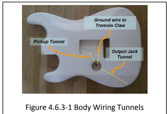
Figure 4.6.3-1 Body Wiring Tunnels
