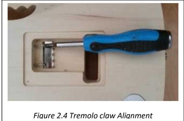
Figure 2.4 Tremolo claw Alignment
